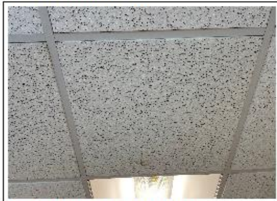
6. Room 2285: Some ceiling tile staining
